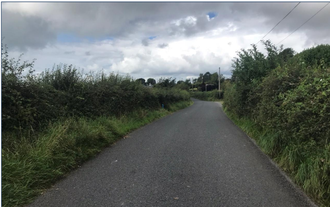
Plate 12-16 Roadside screening existent on the L7001
