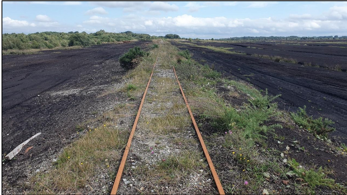
Plate 12-4 Existing conditions at the Application Site, showing the railway track traversing a drained area of cutover bog
